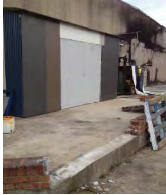
View of the bunded plant area Looking south east
